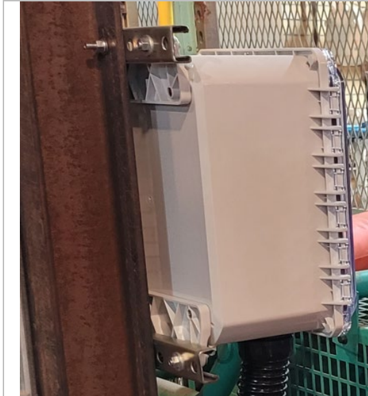
Mounted on beam with Unistrut
