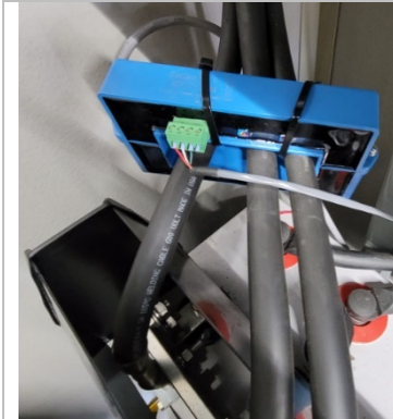
Secure CT with cable ties.
